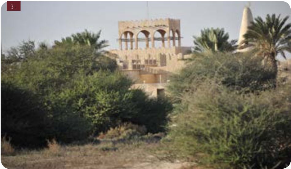
Film city, located in the north of Zekreet where the office of the General Directorate of Natural Reserves is settled
